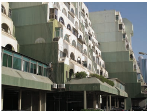
Figure 10. Al-Sawaber complex with façade alterations (photograph by author).
